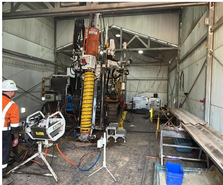
Figure 1 Second diamond drill rig operating inside the acoustic shed at the Blue Moon Target
