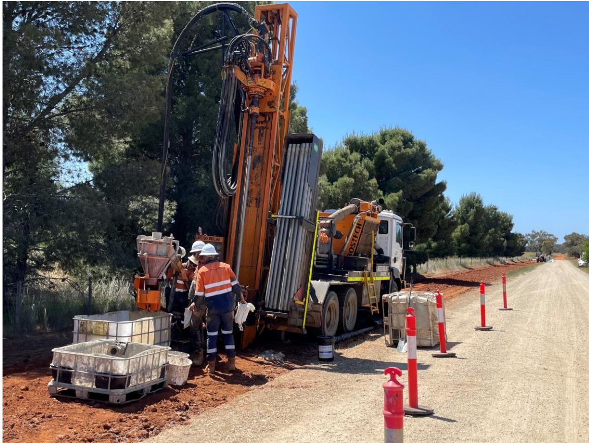
Figure 2 Bostech Aircore Rig Mobilised
