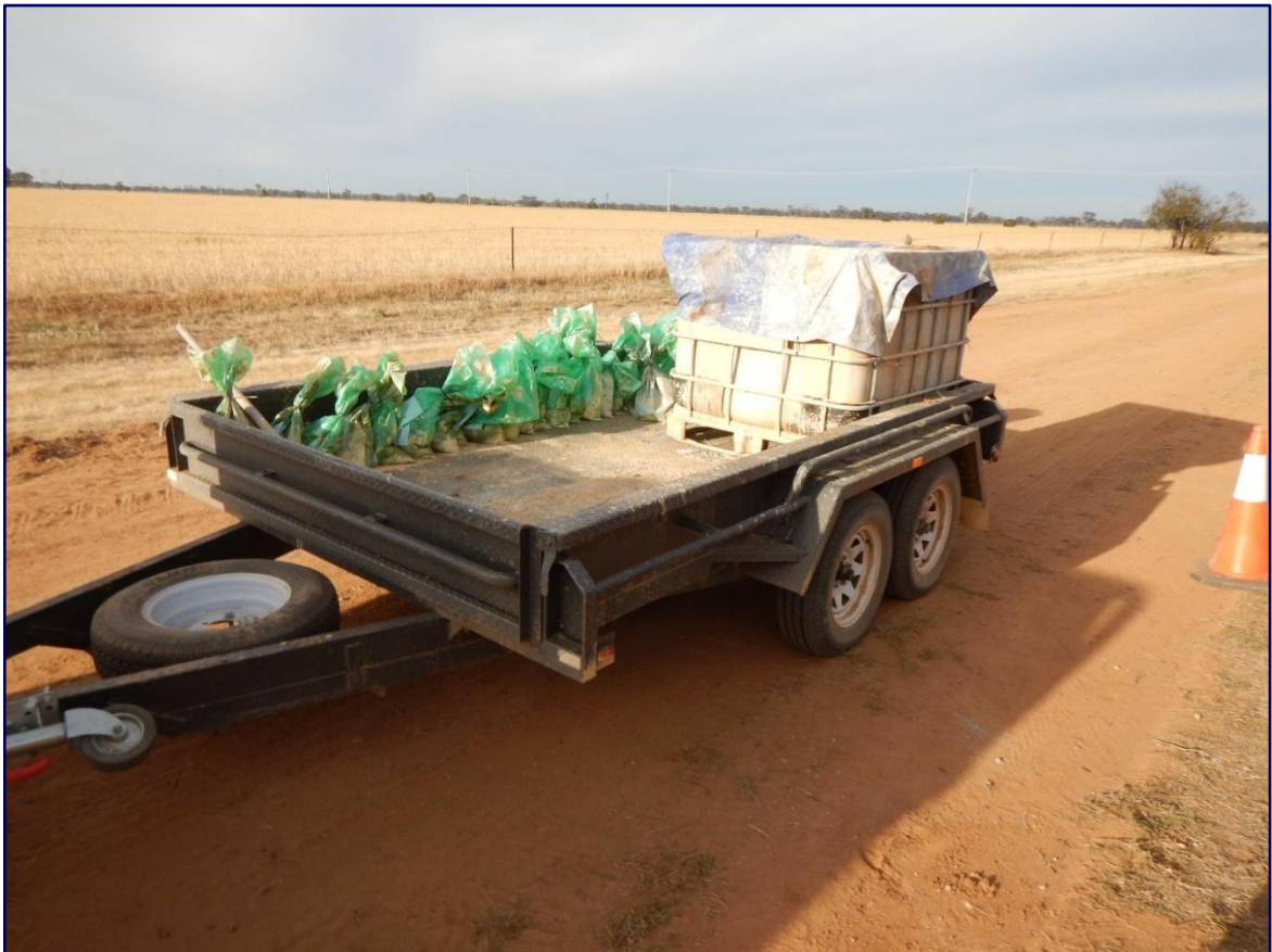
Figure 4 Removal of collected water and waste material
